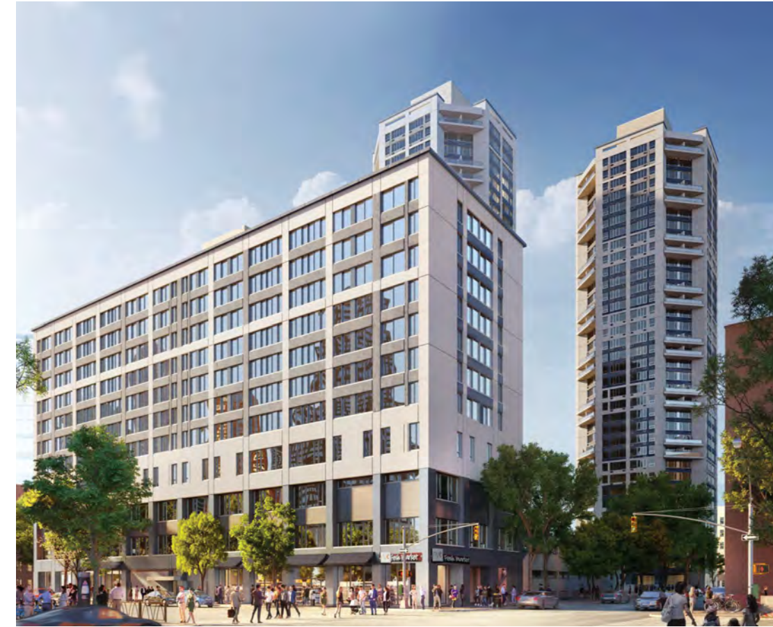
The Heritage is a mixed-use development in Manhattan's East Harlem neighborhood. It is set to undergo improvements to the envelope and the integration of high efficiency heat pumps.
