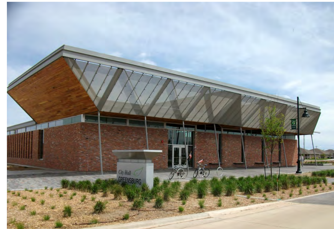
The City Hall building in Greensburg, Kansas, includes solar panels and a ground-source heat pump system that provides heating and cooling.
